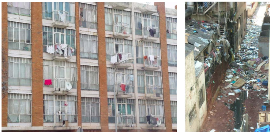
Figure 4.4; Left: poor quality building in Hillbrow, right: trashed alley (Silverman and Zack, 2007)
