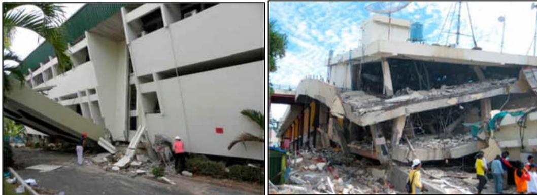
**Figure 4.3** Sinking buildings in Padang due to the soil absorbance effect from earthquake and soil liquefaction in 2009 (Source: EERI, 2009)
