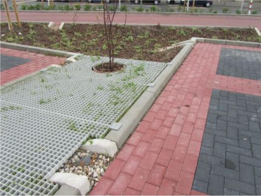
Figure 2.3: Bioretention on unused space of a parking lot in Berlin. Image by Roelofs (2014).
