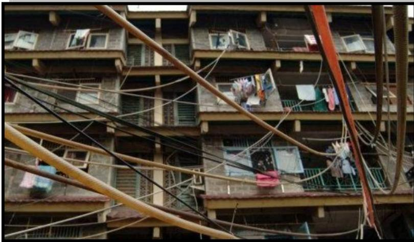
**Figure 4.7** Water hoses from other source because lack of water supply in Rusunawa Merunda, Jakarta
