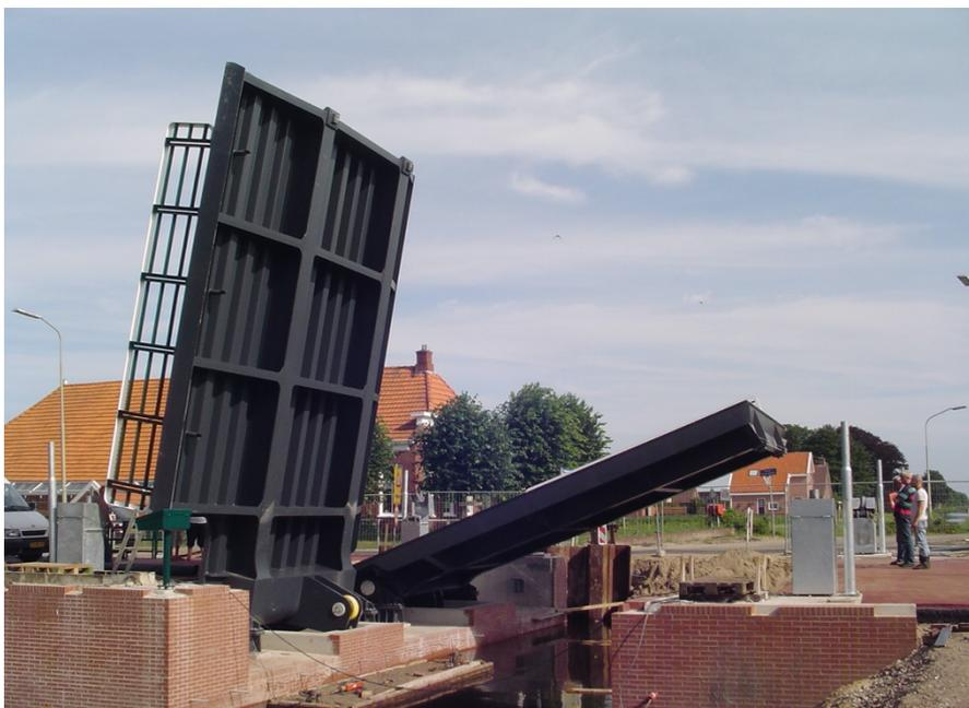
Figure 7: 2006: Central dam in Kiel-Windeweer is replaced by a modern drawbridge. In the background the old dam is still visible (source: [kiel-windeweer.nl](http://kiel-windeweer.nl))
