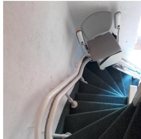
Figure 11: Example of a stair-lift ([trapliften.nl](http://trapliften.nl))
