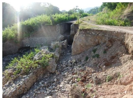
*Figure 11 - Picture of the landslide interrupting Bena main canal*
