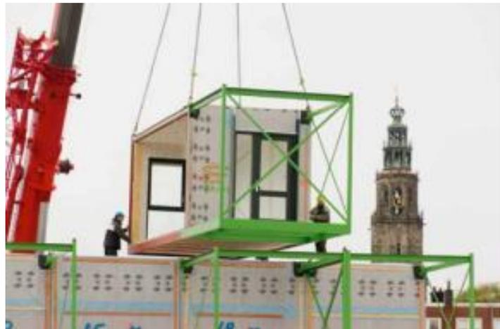
Figure 4.3: pavilion installation (Source: Bervoet & Van Tuijl, 2013)
