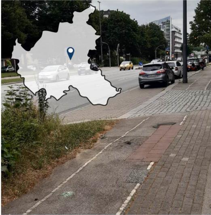
Figure 10. Narrow bicycle path with bad surface and broken glass next to four lanes of motorised traffic. Hamburg, Eiffestraße. Own image.
