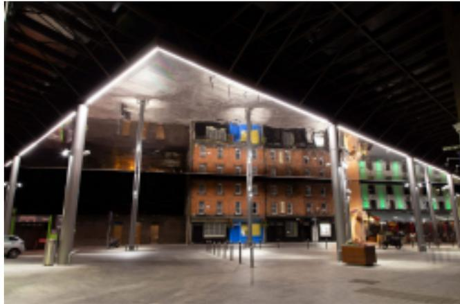
Fig (13): The Apple Market, Waterford City located at John Street. It is a 1 400 m<sup>2</sup>, 9 m-high, triangular glass and steel canopy structure which was part of Waterfords urban regeneration scheme (Dlight, 2021).
