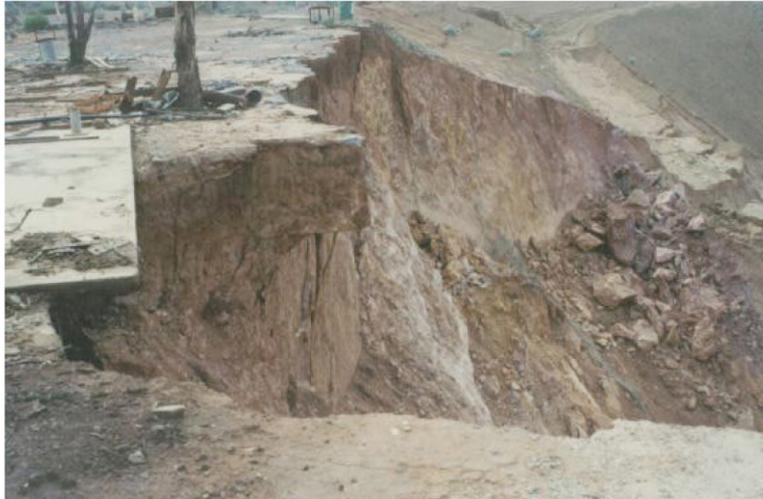
Figure 2.1 Progressive long-term failure of a slope in open pit
