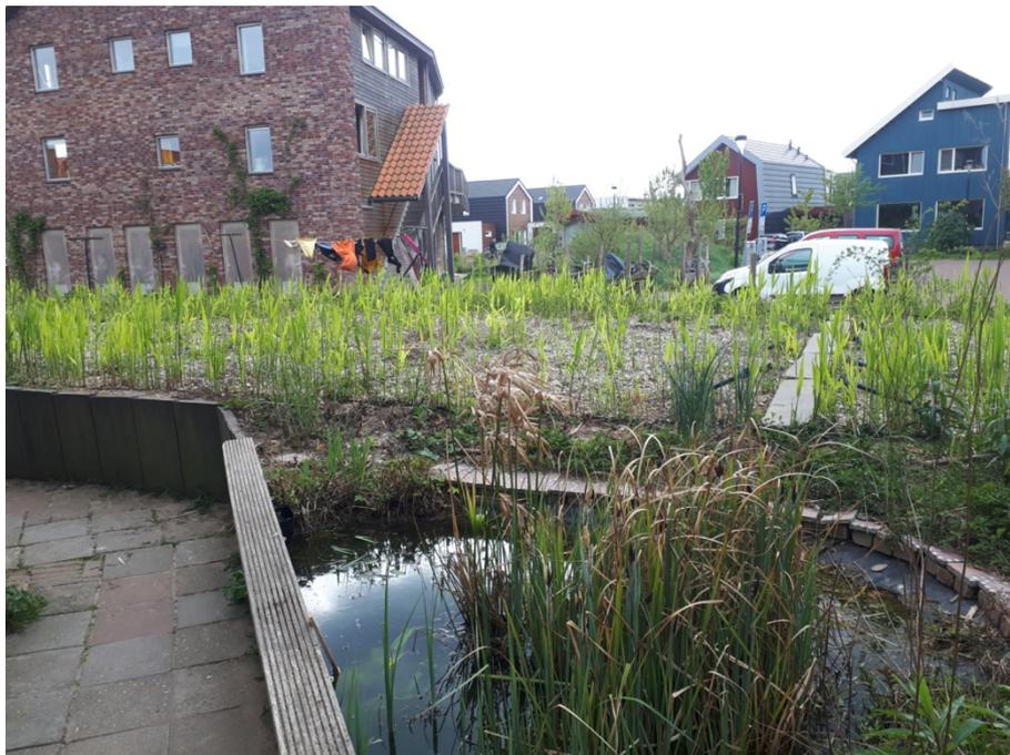
**Figure 7:** Halophyte water-filter system in IEWAN. Gray water from IEWAN is filtered via this system and re-used to flush toilets.
