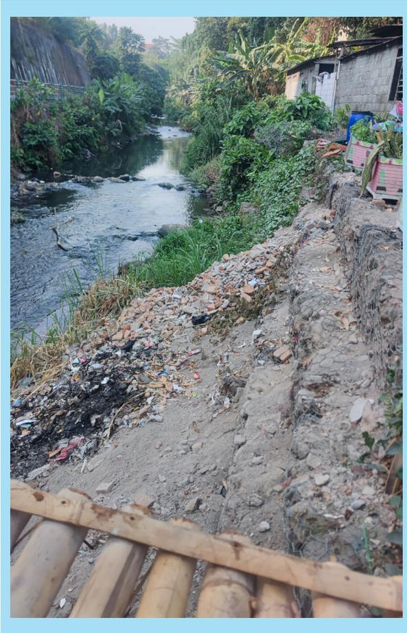
**Fig. 4.6.** A part of the dyke in Caturtunggal that has not been completely reinforced yet.
