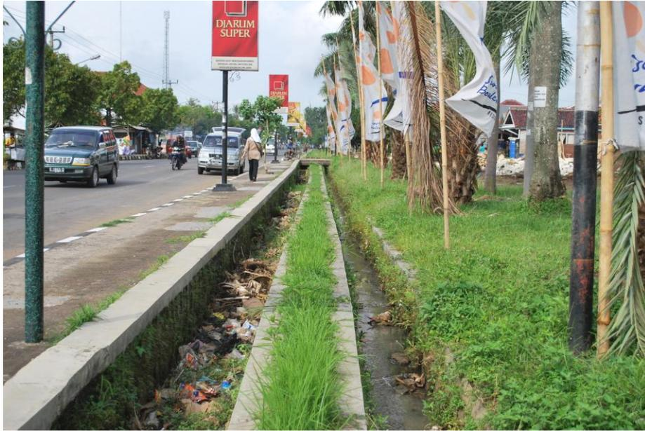
**Figure 4.13** Drainage system condition in front of the ‘*Sunrise Boulevard*’, a large middle class real estate in the District of Cirebon
